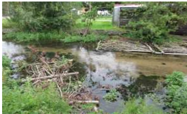
Deflectors at Walsworth Common
